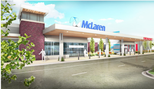
McLaren Health – West Branch, MI Health system owned, big box retail store redeveloped into ambulatory care center.
