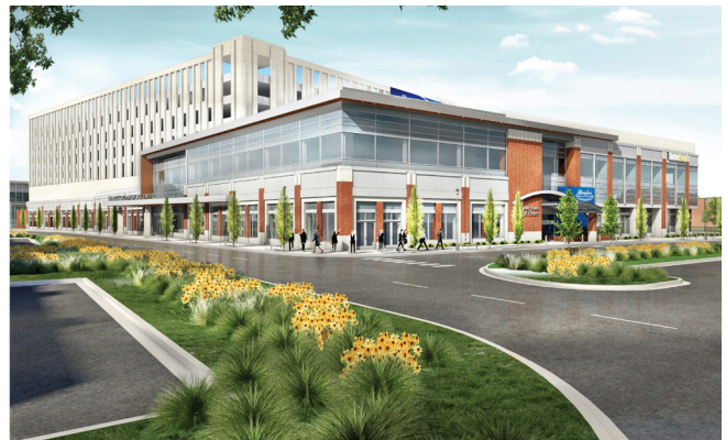
Henry Ford Health - Bloomfield, MI redevelopment came with an attached parking structure serving the campus development
