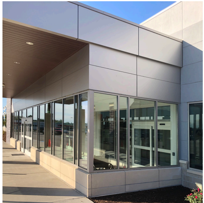
New entrance canopy and vestibule
